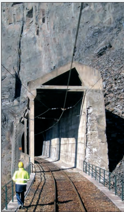
Figure 6 - The 1921 protective gallery with the tunnel in the background.
