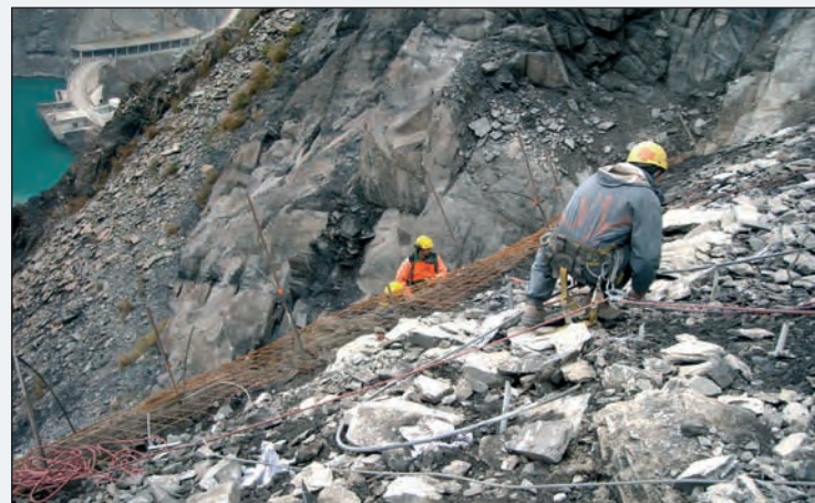
Figure 10 - Exceptional working conditions at the tunnel head (waterproofing injection).
