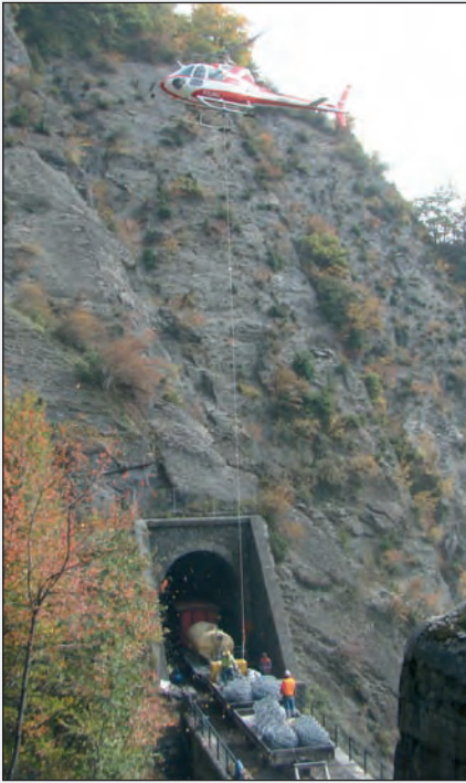
Figure 8 - Supply of the worksite by train and installation by helicopter.
