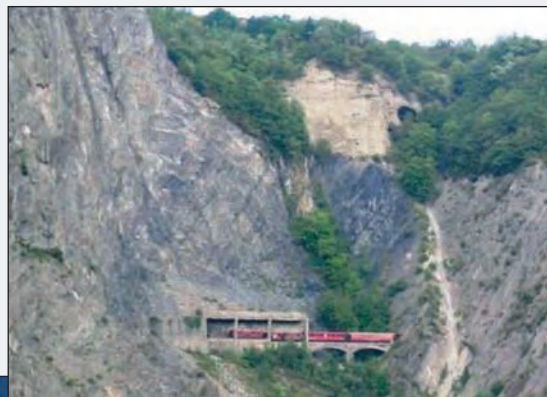
Figure 4 - View of the tunnel head, the protective gallery and the Clapisse viaduct from the opposite bank of the Drac.
