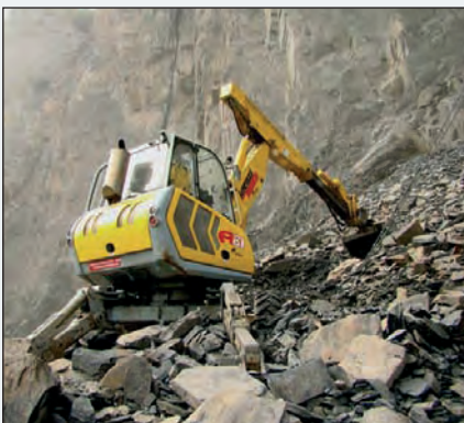
Figure 9 - Work on scree using walking excavator.
