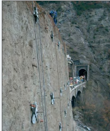
Figure 13 - Strengthening the downside side wall.
