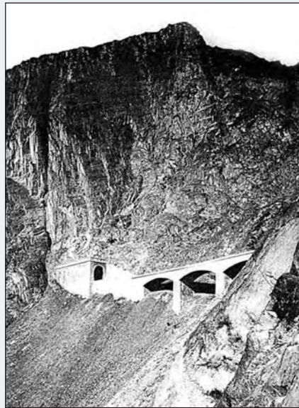
Figure 3 - Southern tunnel head and the viaduct as they were between 1894 and 1921.
